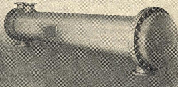
Brine to brine heat exchanger, all internal construction is stainless steel. Size 20" x 10'.
